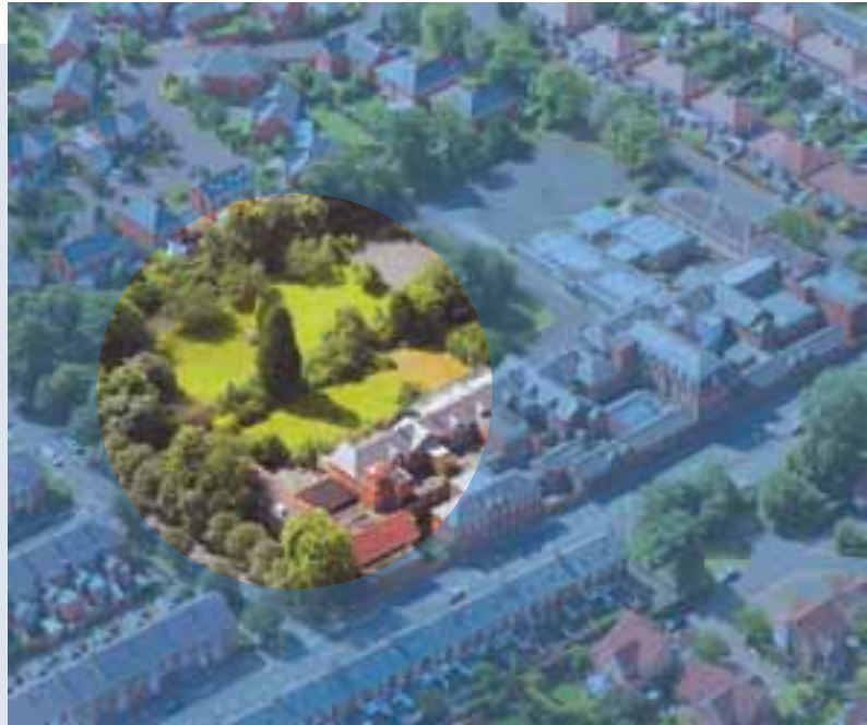
Site of the proposed Gosforth Healthcare and Treatment Centre serving the north of Newcastle
