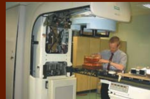
Northern Centre for Cancer Treatment: delivery of new Linear Accelerator
