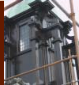
Refurbishment of the RVI lantern tower
